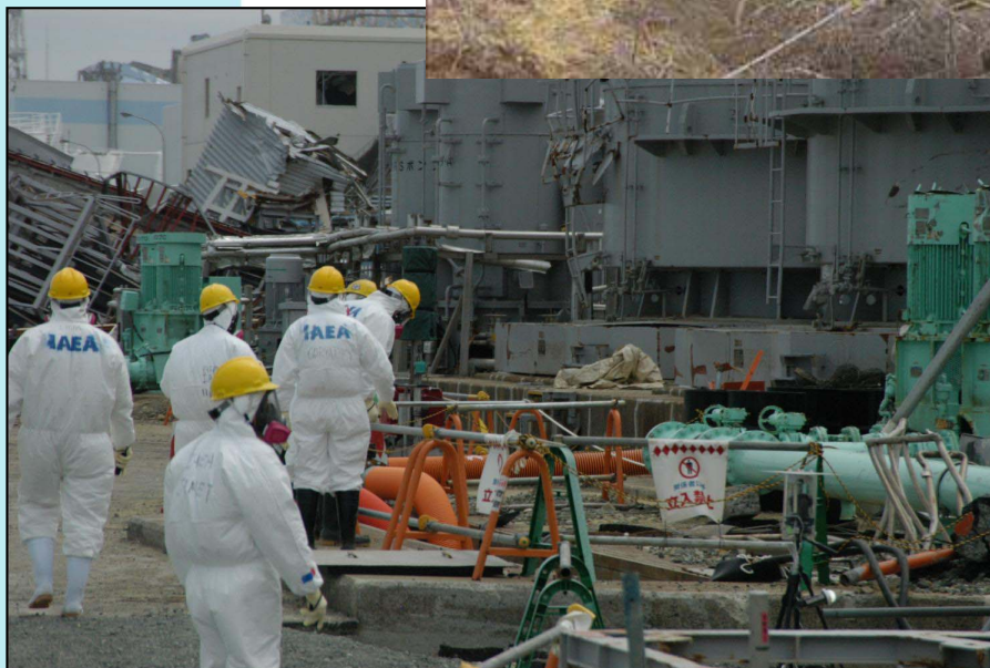
Damage of back-up power sources
